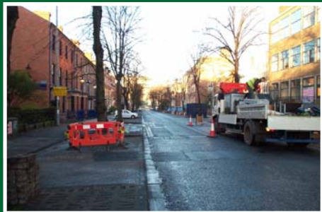
Minimal Disruption being caused Pipe Bursting on Elmwood Avenue, Belfast
