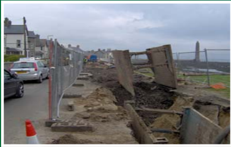
Disruption caused by Typical Trenched Installation
